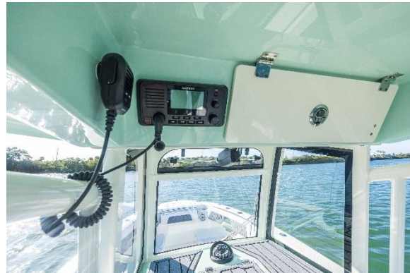
Forward Electronics Storage
