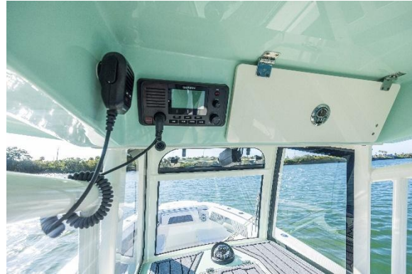
Forward Electronics Storage
