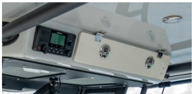
Forward Electronics Storage
