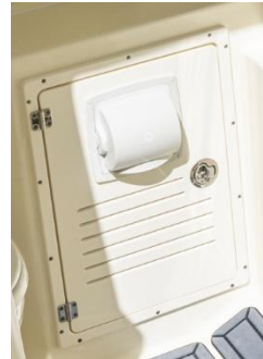
House Battery Access
